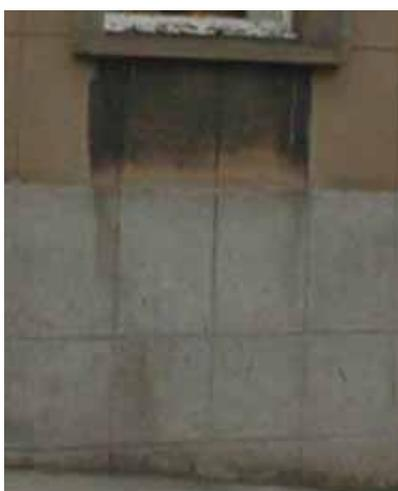
Impermeable render showing signs of water retention within the wall.
