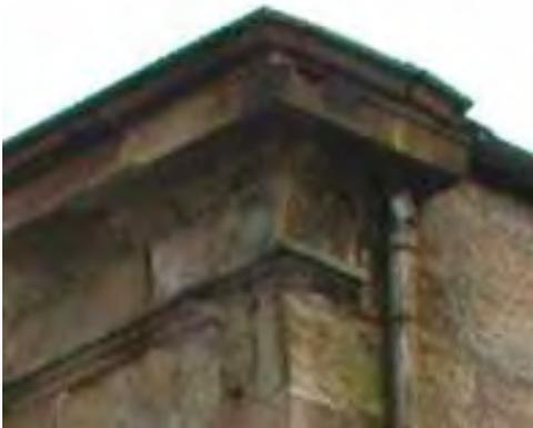
Faulty drainage from this roof is causing damage to the ashlar.
