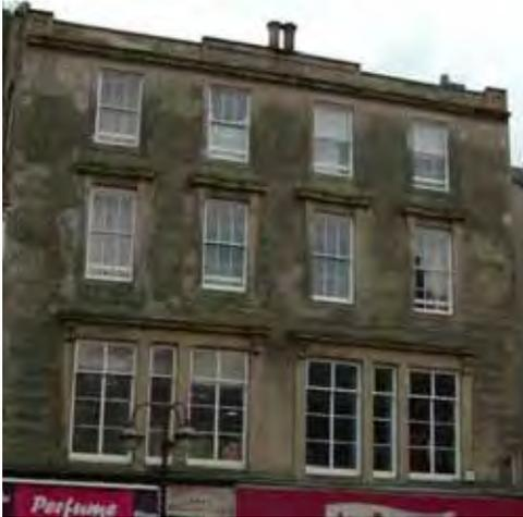
105-111 High Street, where the masonry is appears to be saturated
