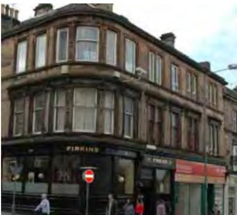
Window replacement on the second floor of 42 Vicar Street. Note the filled-in window on the corner (ground floor).
