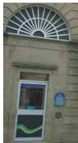
The aluminium door is inappropriate for this A-listed building.
