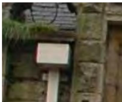
Vegetation growing in the gutter; replacement downpipe square profile, unlikely to match the original. The building is C(S) listed.
