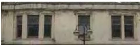
Rainwater goods and paint are in poor condition.
