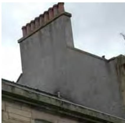
Impermeable render to chimney and gable, likely to cause problems for evaporation of moisture.
