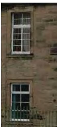
Original windows at upper level, uPVC replacements at ground level. Neither the material nor the pattern of the new matches the original. This is a listed building.
